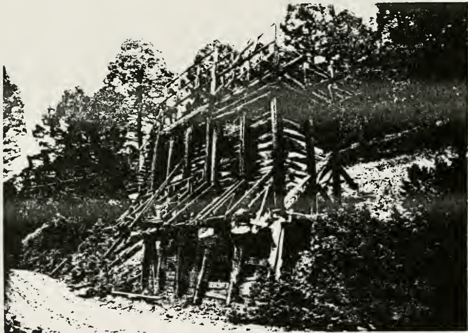
Figure 254. Feature #151, ore bins, northeast view.
